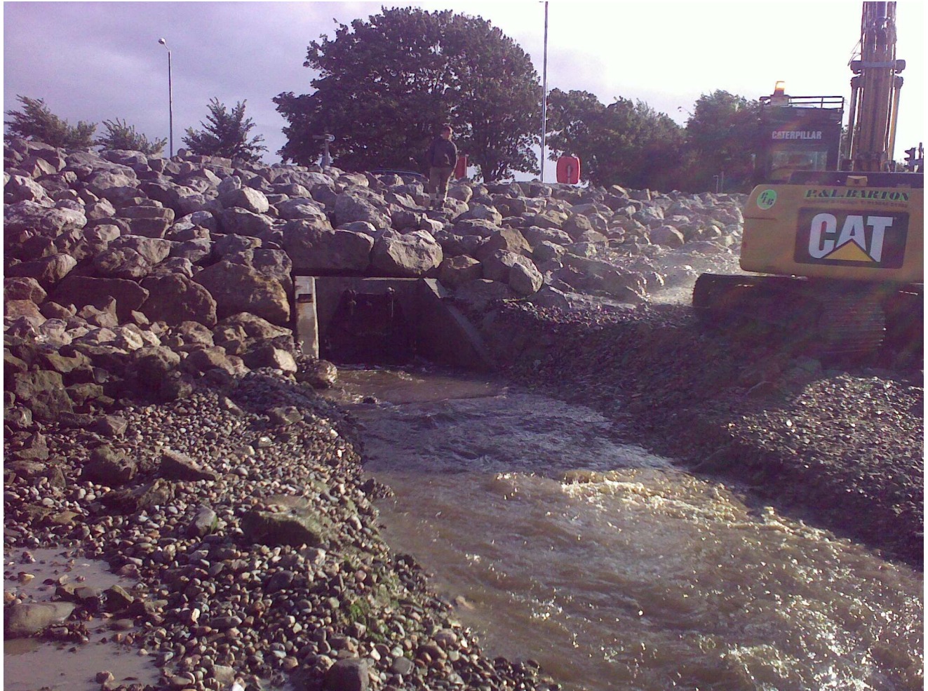
Bare Beck outfall after clearance.
